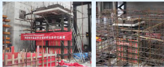
Cyclic and shaking table tests of rocking pile-group foundation
